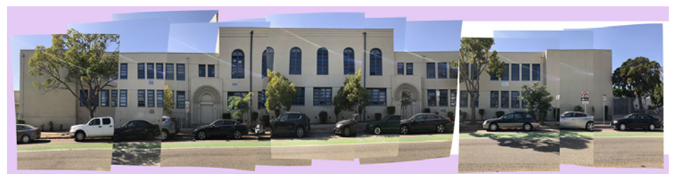
The English Building at Santa Monica High School. 7th Street Elevation composite: Nina Fresco
