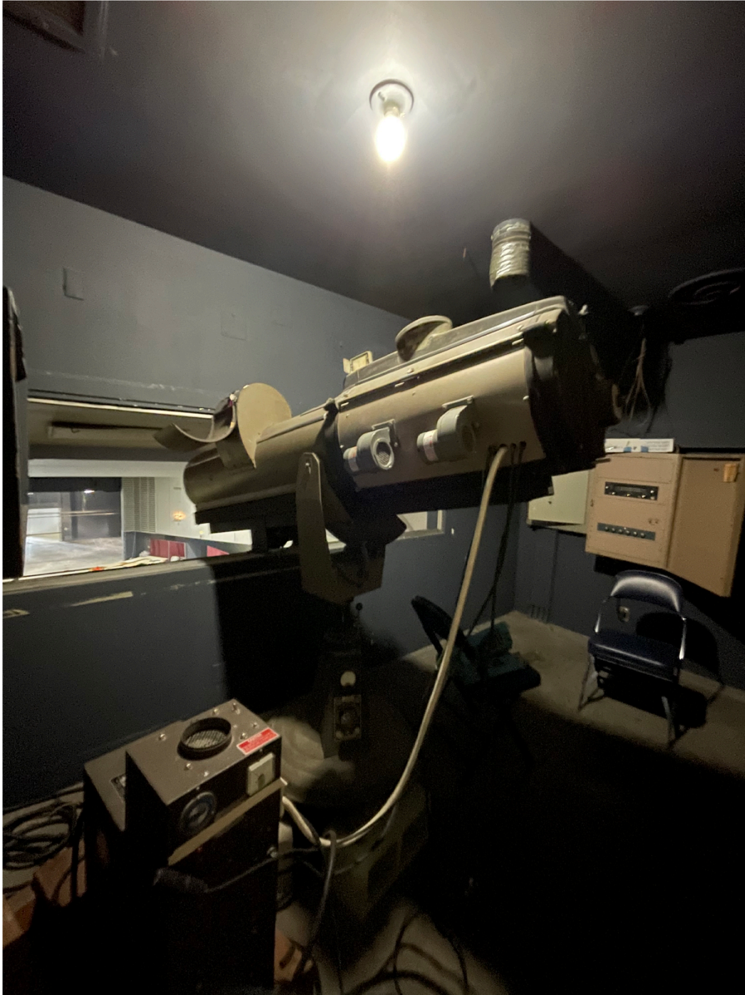
Figure 29. Spotlight inside 4th floor projection booth (view south). Image: Nina Fresco, 2023
