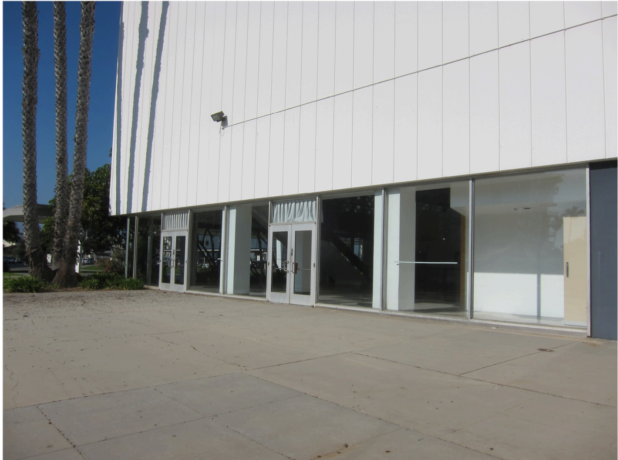
Figure 12. West Patio, scored concrete volume over glass-enclosed lobby (view north). Image: Nina Fresco, 2014
