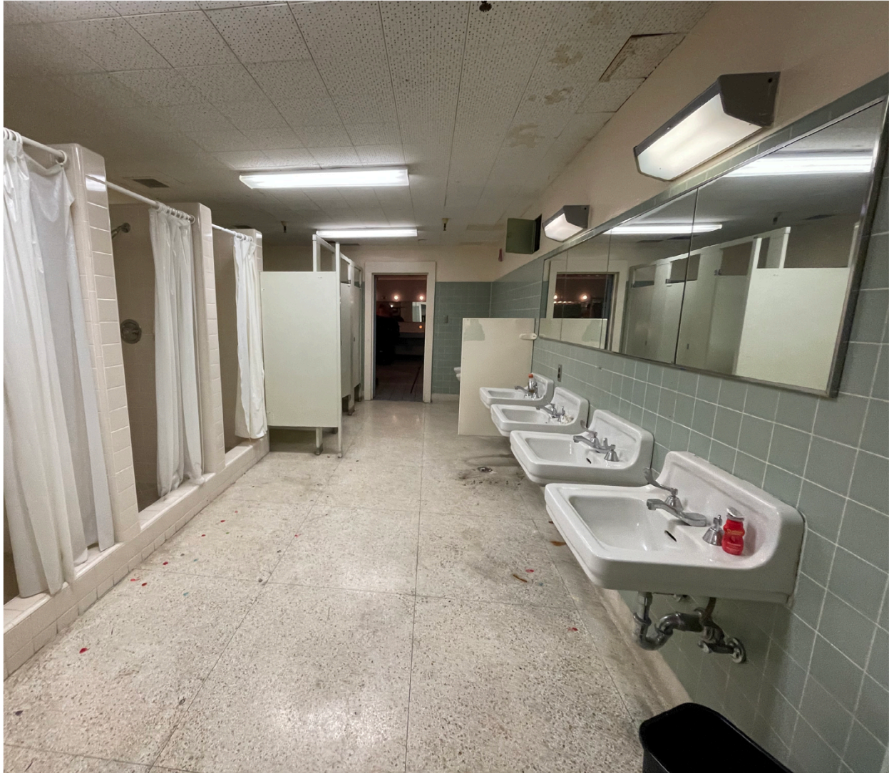
Figure 30. Dressing room, original bathroom tile and fixtures (view northwest). Image: Nina Fresco, 2023
