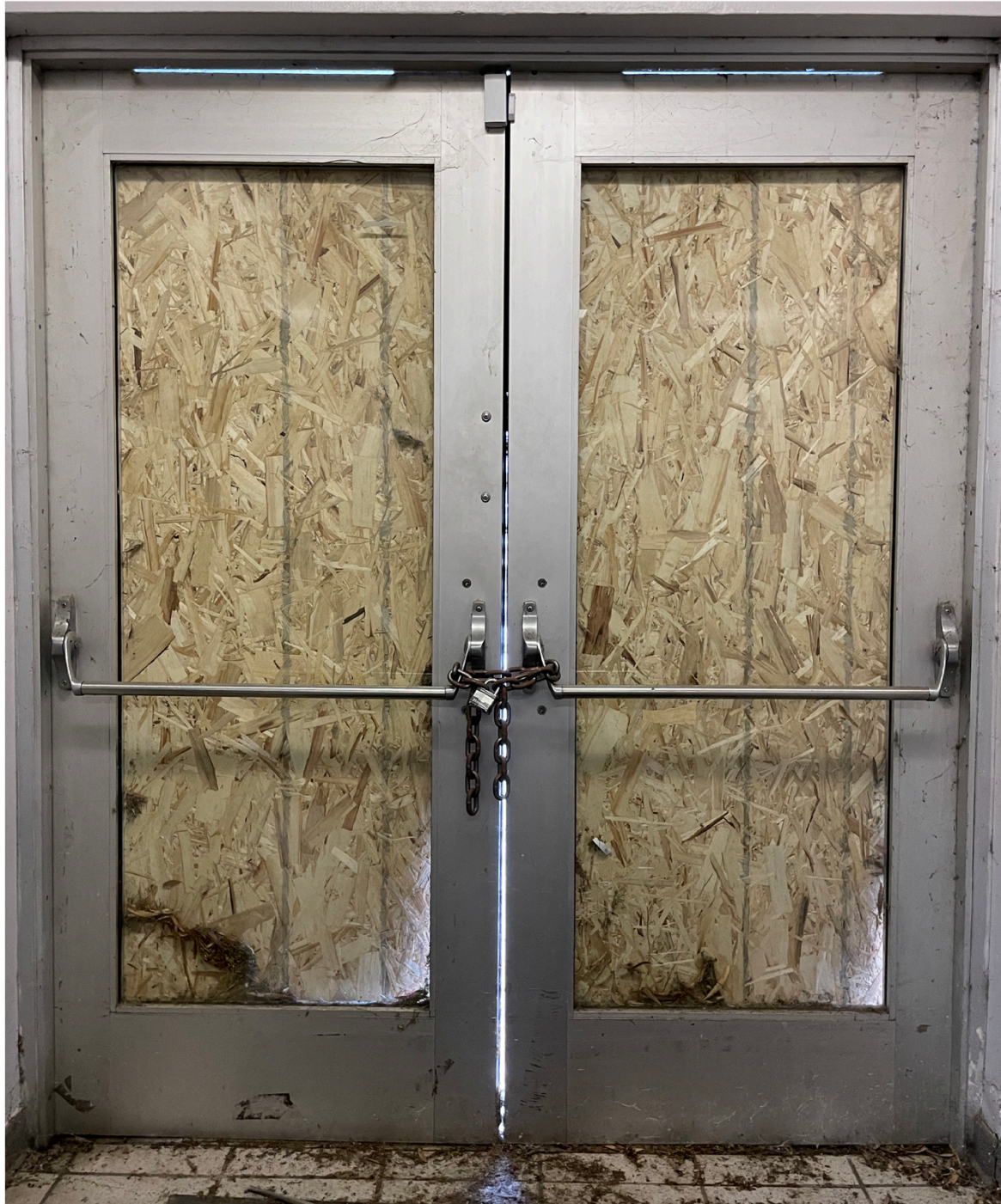
Figure 14. East Wing, framing and hardware of typical entry door (view northeast, from interior hallway, east wing). Image: Nina Fresco, 2023
