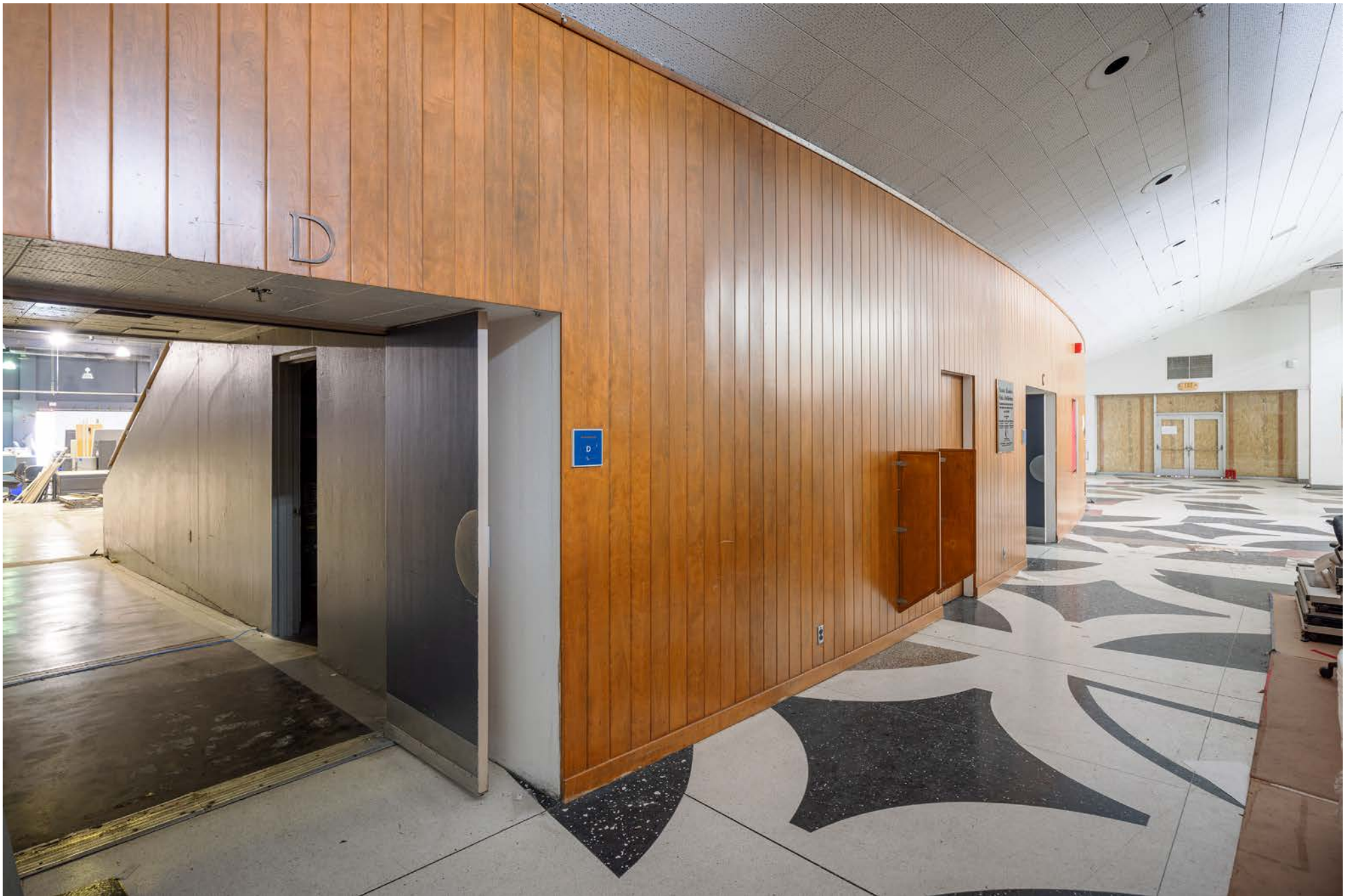
CA_LOS ANGELES COUNTY_SANTA MONICA CIVIC AUDITORIUM_0013.TIF INTERIOR MAIN LOBBY: VOMITORIUM AND HINGED FLOOR (LEFT), CURVED LOBBY VOLUME (RIGHT), CAMERA FACING SOUTH.
