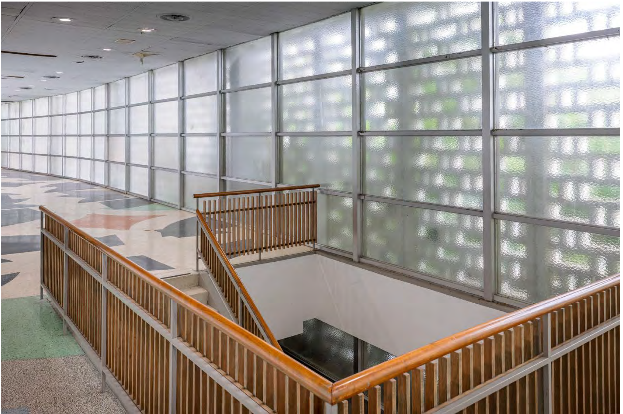
CA_Los Angeles County_Santa Monica Civic Auditorium_0014.tif INTERIOR UPPER LOBBY: NORTHWEST/PRIMARY ELEVATION (LEFT), CAMERA FACING WEST.
