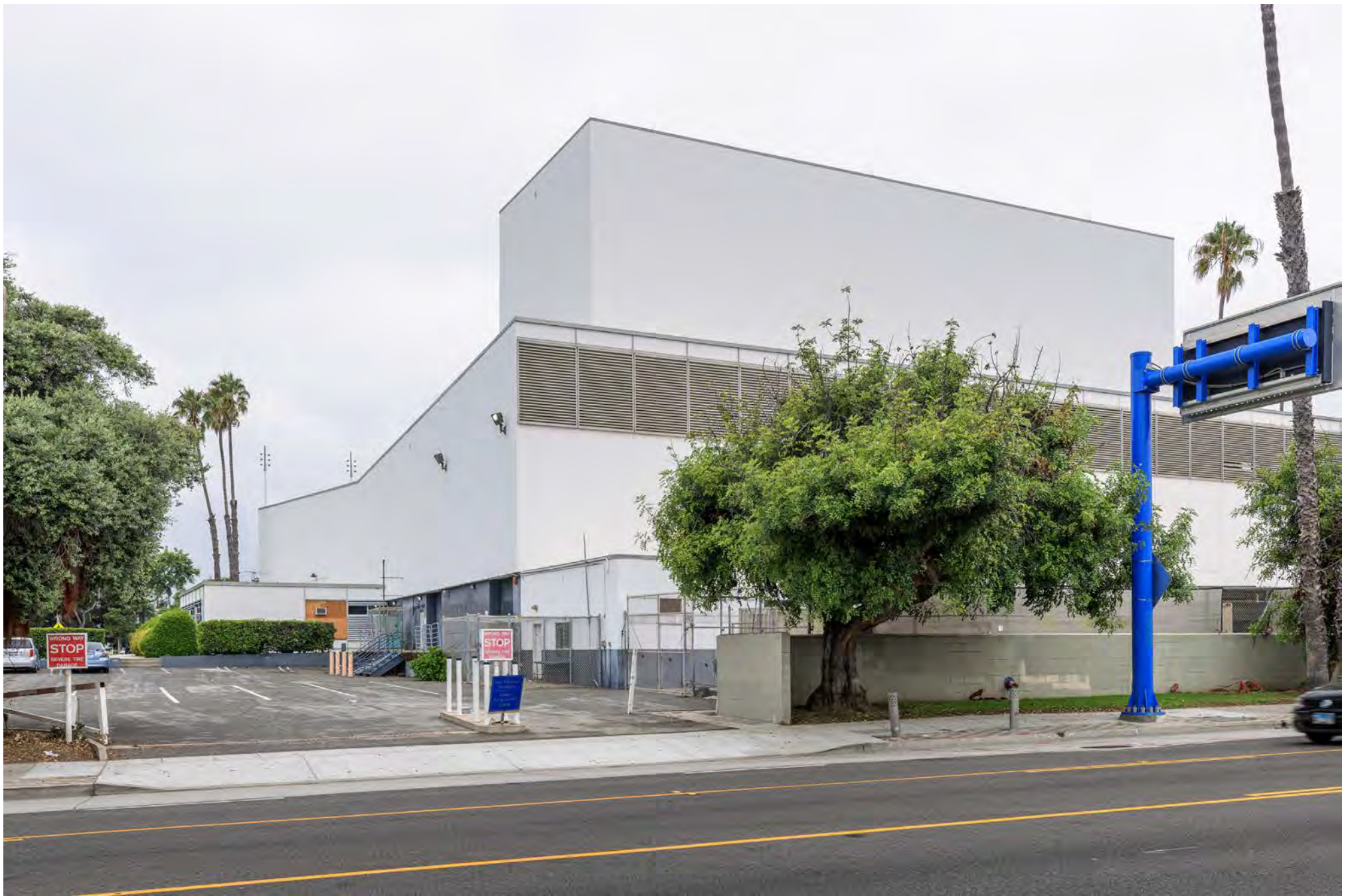
CA_LOS ANGELES COUNTY_SANTA MONICA CIVIC AUDITORIUM_0006.TIF SOUTHEAST/REAR ELEVATION (RIGHT), SOUTHWEST ELEVATION AND WEST WING (LEFT), CAMERA FACING SOUTH.
