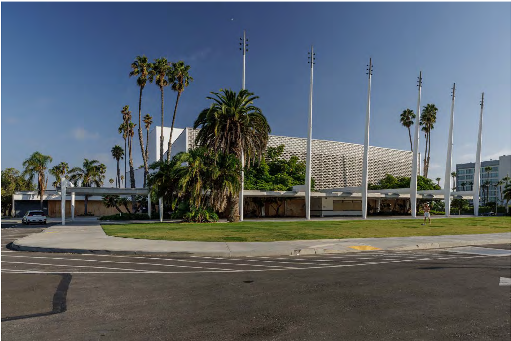
CA_LOS ANGELES COUNTY_SANTA MONICA CIVIC AUDITORIUM_0002.TIF NORTHWEST/PRIMARY FAÇADE (RIGHT), EAST WING (LEFT), CAMERA FACING SOUTH.
