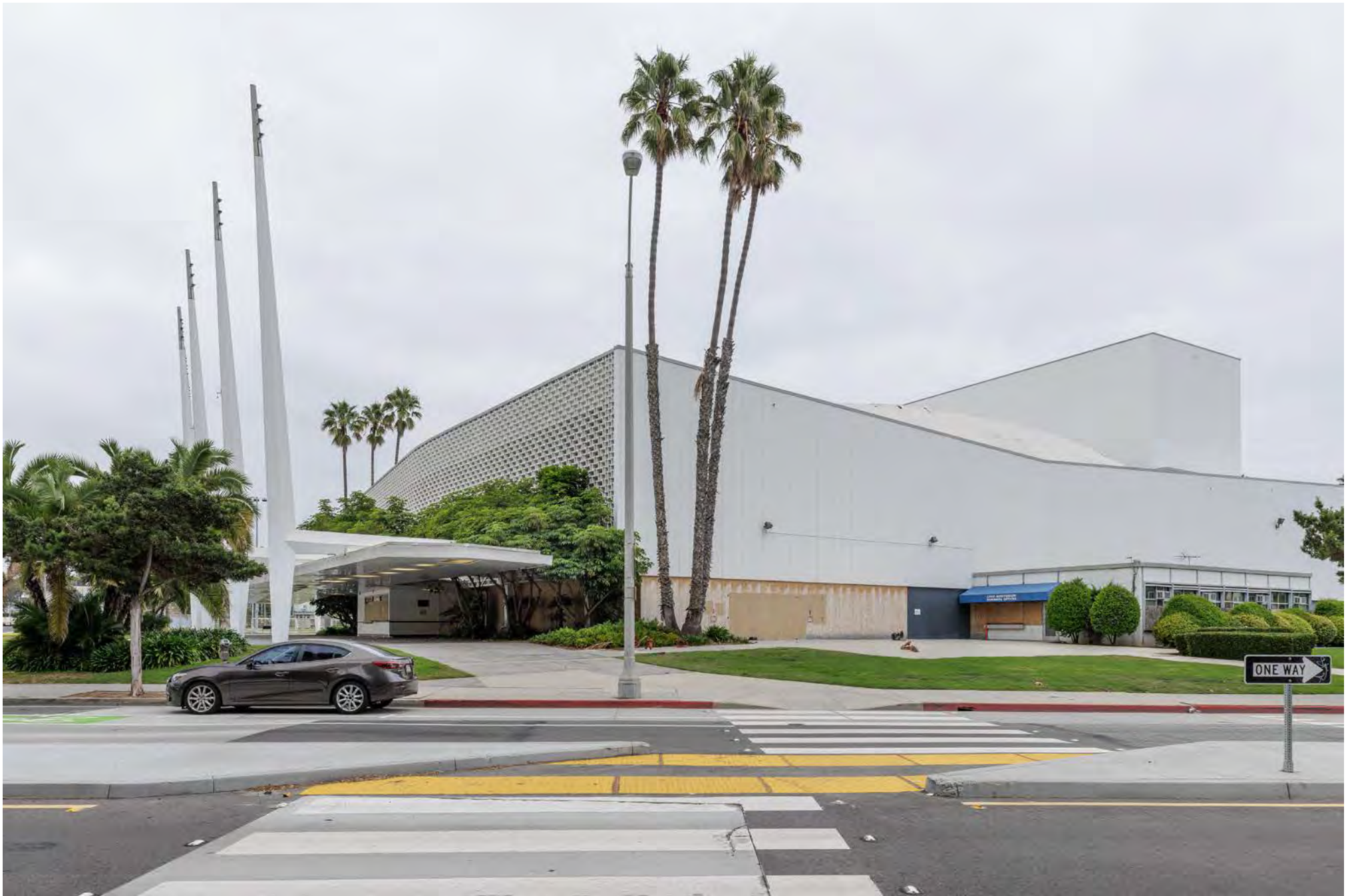
CA_LOS ANGELES COUNTY_SANTA MONICA CIVIC AUDITORIUM_0009.TIF NORTHWEST/PRIMARY FAÇADE (LEFT), SOUTHWEST ELEVATION AND WEST WING (RIGHT), CAMERA FACING EAST.
