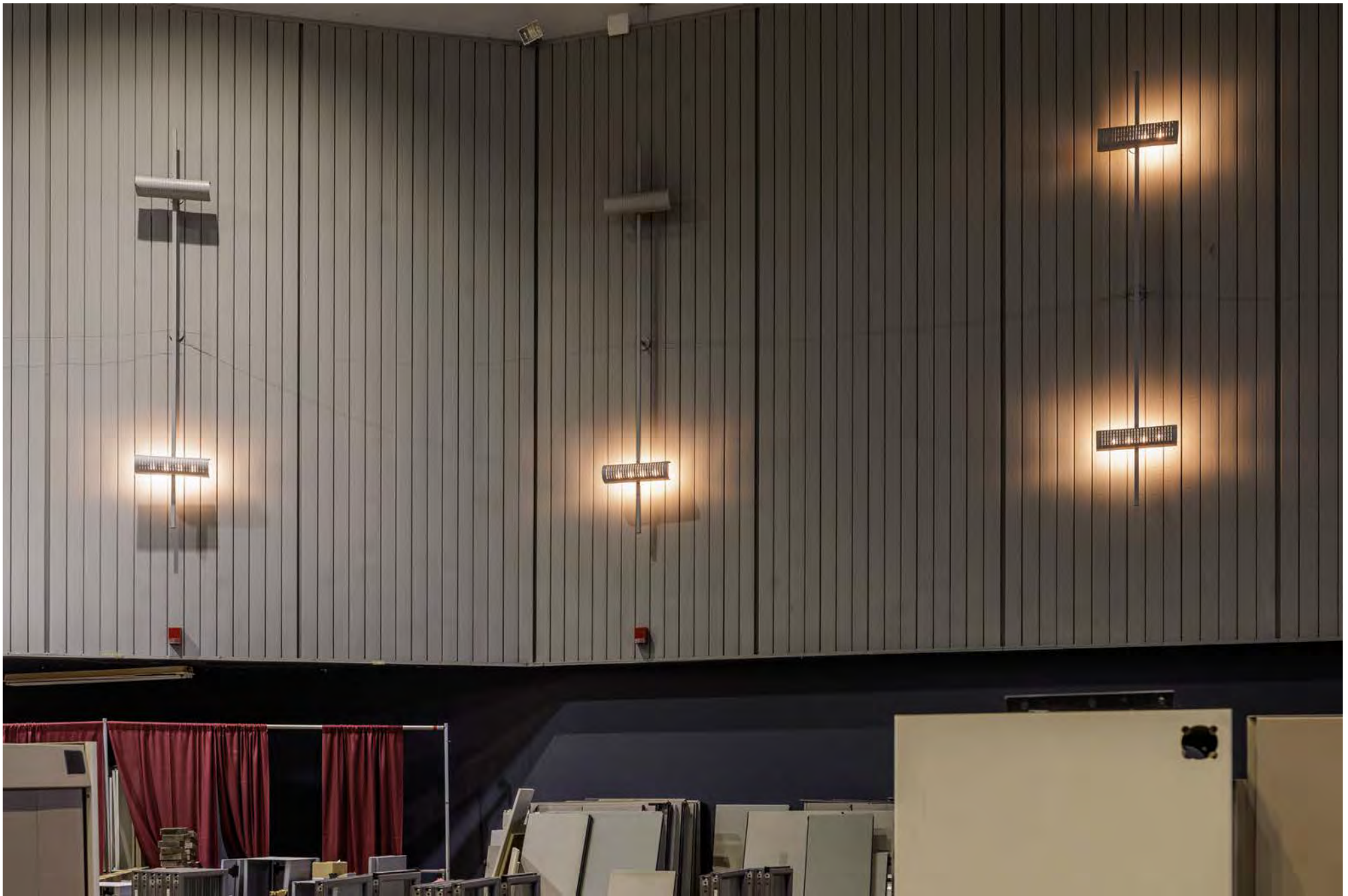
CA_LOS ANGELES COUNTY_SANTA MONICA CIVIC AUDITORIUM_0020.TIF INTERIOR AUDITORIUM, DETAIL: METAL ACOUSTIC PANELS AND CUSTOM SCONCES, CAMERA FACING NORTH.
