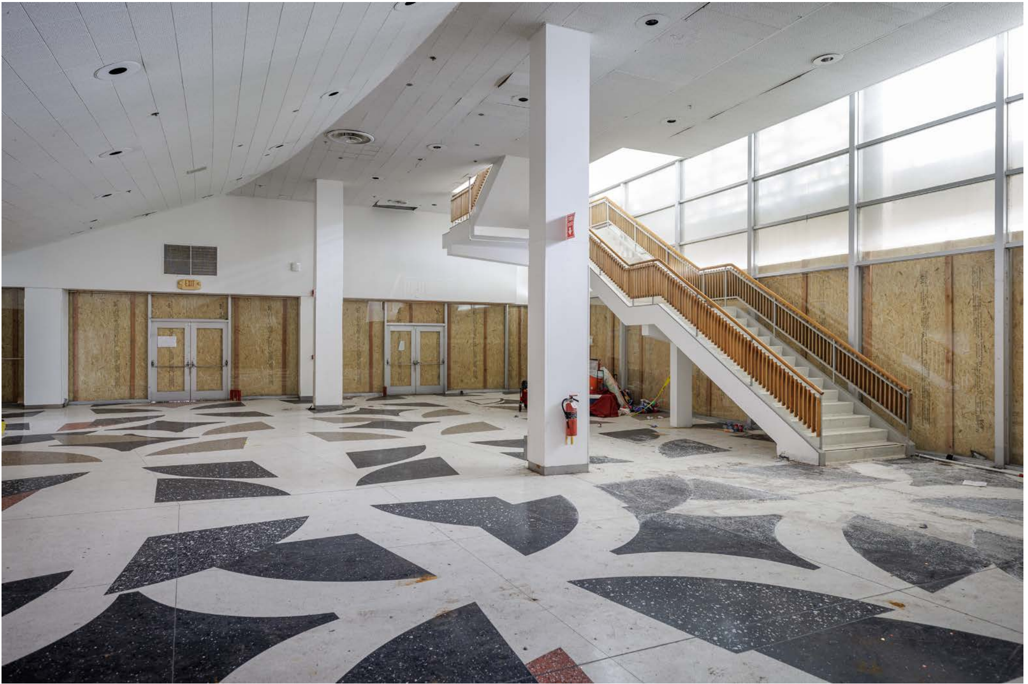
CA_LOS ANGELES COUNTY_SANTA MONICA CIVIC AUDITORIUM_0012.TIF INTERIOR MAIN LOBBY: STAIR AND NORTHWEST/PRIMARY FAÇADE (LEFT), CAMERA FACING WEST.
