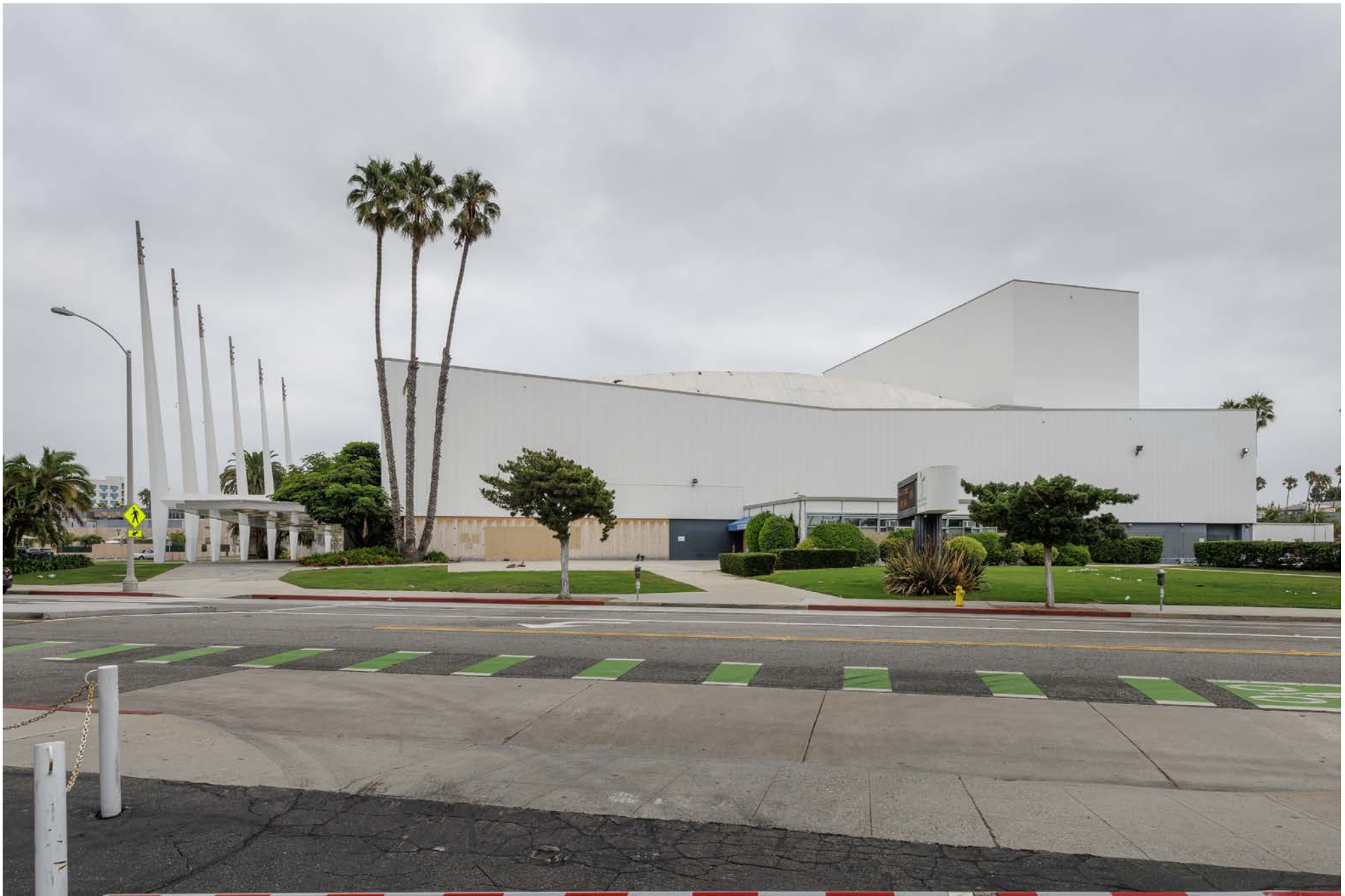
CA_LOS ANGELES COUNTY_SANTA MONICA CIVIC AUDITORIUM_0008.TIF SOUTHWEST/REAR ELEVATION AND WEST WING (RIGHT), FAÇADE CANOPY AND PYLONS (LEFT), CAMERA FACING NORTHEAST.
