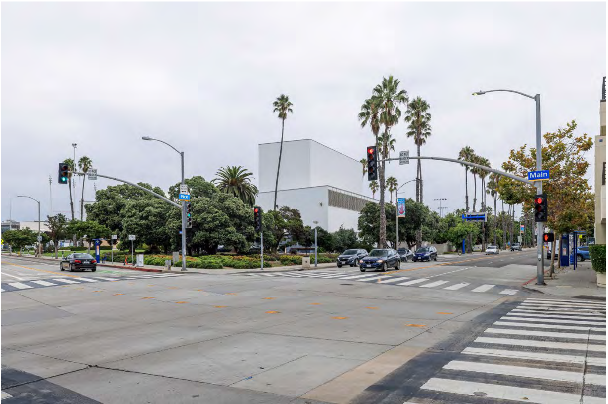
CA_LOS ANGELES COUNTY_SANTA MONICA CIVIC AUDITORIUM_0007.TIF SOUTHEAST/REAR ELEVATION (RIGHT), SOUTH BOUNDARY BELMAR NEIGHBORHOOD (FOREGROUND), CAMERA FACING NORTH.
