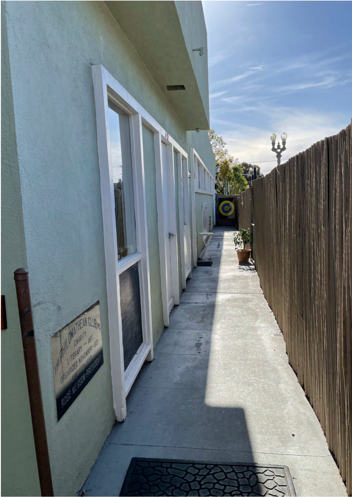
Philomathean Club Building, Oblique view of north-facing facade. February 2023
