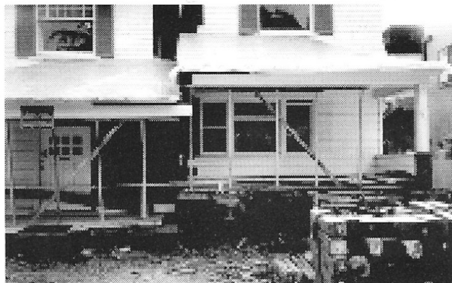
The house had to be split to be moved.
