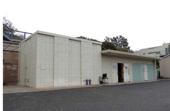
Old Utility Building (U), 1960. Southeast view.
