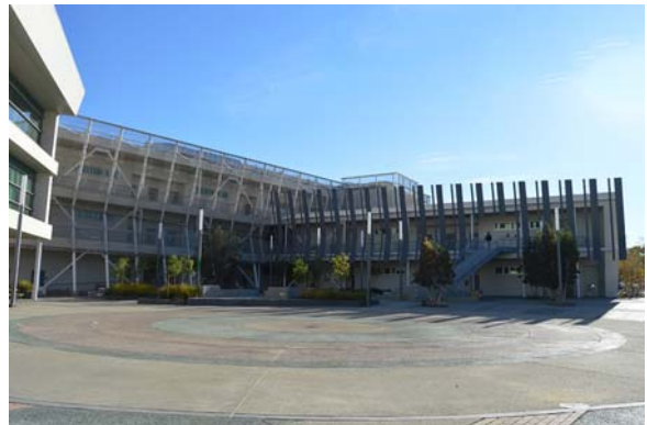
Innovation Building (I), 2015. Southeast view (from Centennial Quad).
