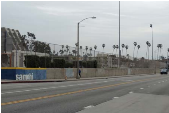
West perimeter. Southeast view.
