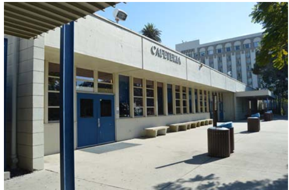
Cafeteria (K), 1960. Southeast view.
