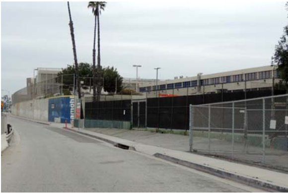
North perimeter. Southeast view.
