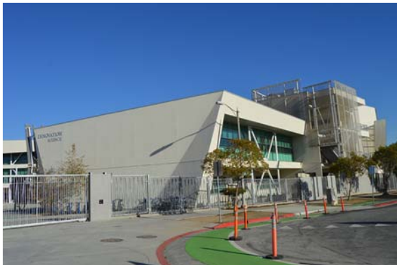
Innovation Building (I), 2015. Northeast view (from Michigan Avenue).
