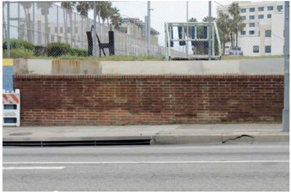
Brick Wall, 1913. North view.
