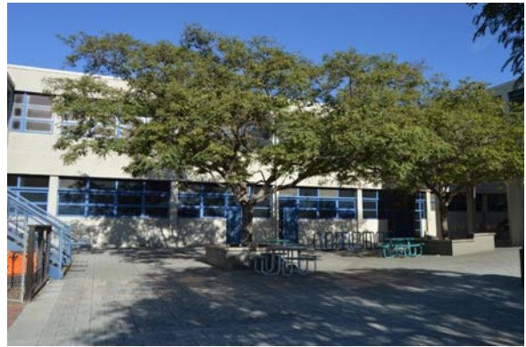
Technology Building (A), 1960. North view (from Science Quad).
