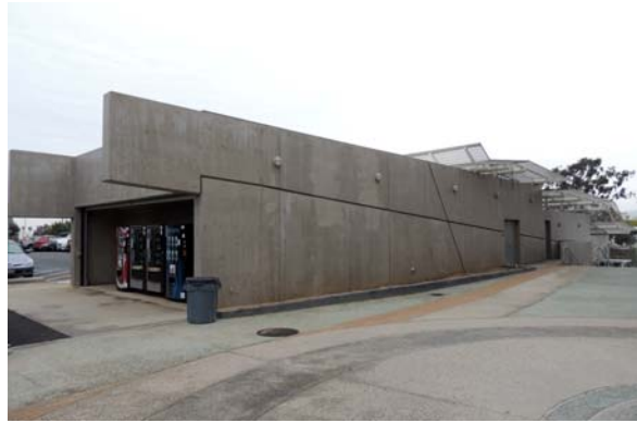
New Utility Building (S), 2016. Northwest view.
