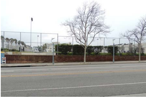
Brick Wall, 1913. North view.
