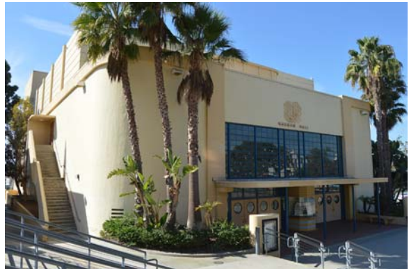
Barnum Hall (H), 1938. Northwest view
