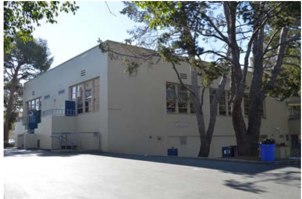
Art Building (E), 1937. Southwest view.
