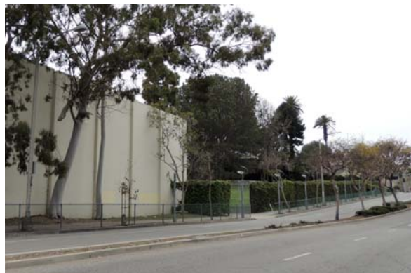
South perimeter. Northeast view.
