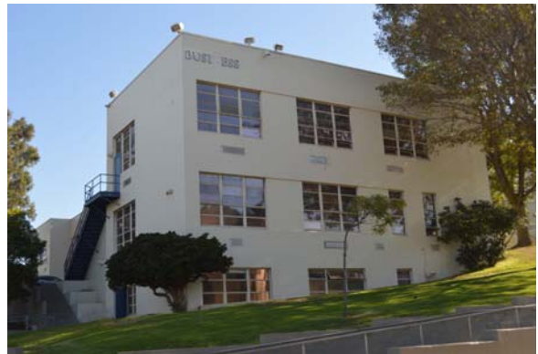
Business Building (C), 1913. East view.
