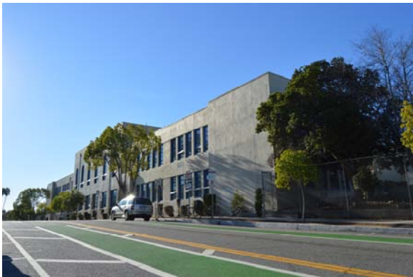
East perimeter. Southwest view.
