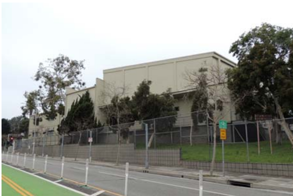
South perimeter. Northwest view.
