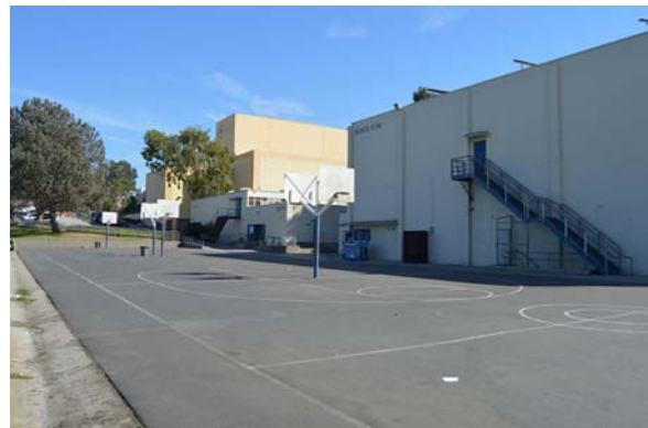
Basketball Courts, c. 2003. Southeast view.
