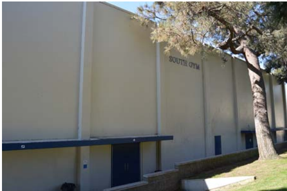
South Gym (P), 1960. Northwest view.
