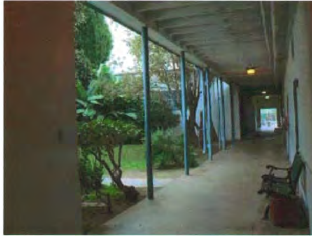
Plate 97. View Along Hallway Toward Playground With Interior Courtyard on Left
