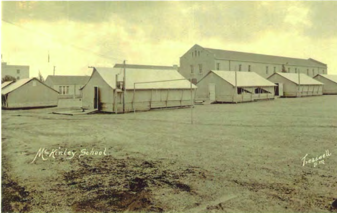
Plate 26. McKinley School, View to Southeast, Showing Tents Set up Behind the School After the March 10, 1933 Earthquake.
