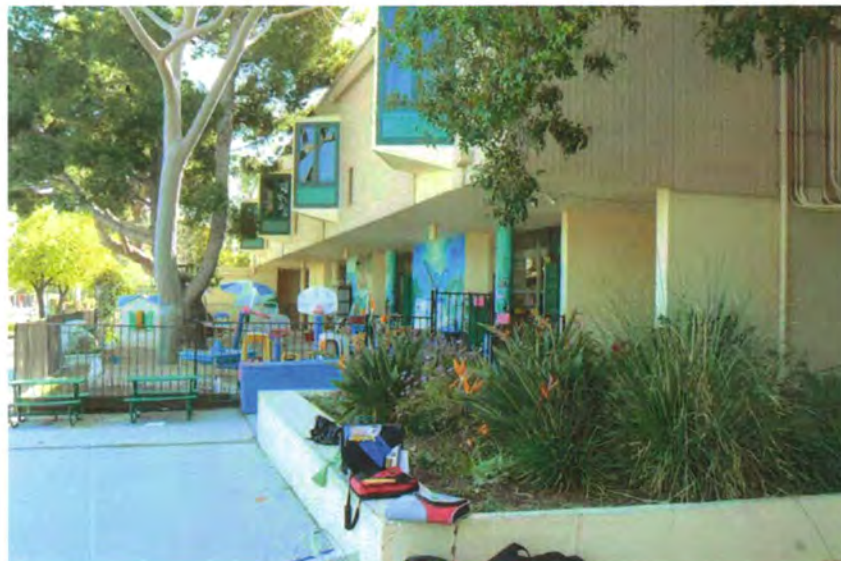
Plate 168. Classroom Building Showing Cantilevered Second Floor, Pilotis, and Projecting Window Diagonals
