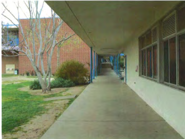
Plate 149. Cantilevered Roof Over Hall in Front of Original Classroom (1963)
