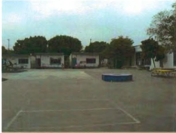
Plate 101. Temporary Classrooms on Playground
