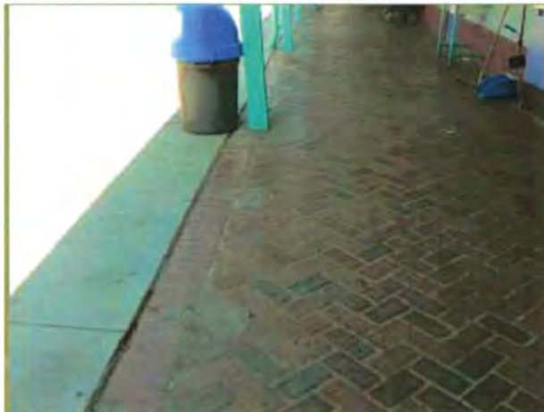
Plate 44. Remnants of Cloister Paving and Column Footings.
