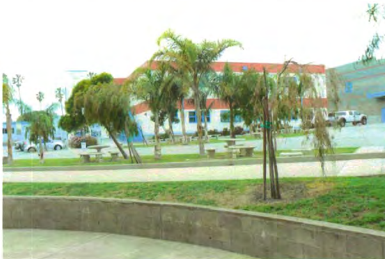
Plate 162. View from Malibu High Main Campus Toward Juan Cabrillo Showing New Classroom and Gymnasium Additions Constructed in Former Parking Area, View to West
