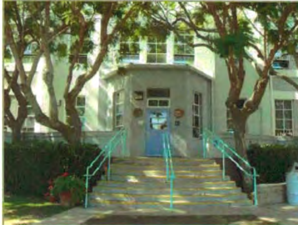
Plate 43. Original Main Building, Lincoln Middle School
