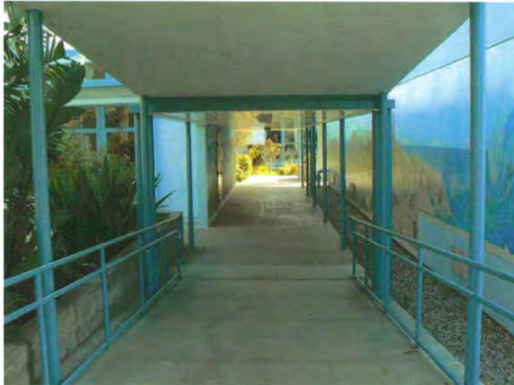
Plate 130. Hallway Connecting Classroom Buildings at West End
