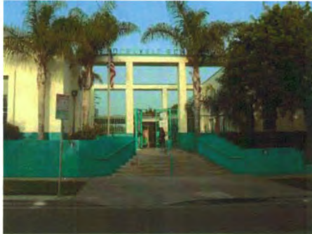
Plate 52. Front Entrance, Roosevelt Elementary School
