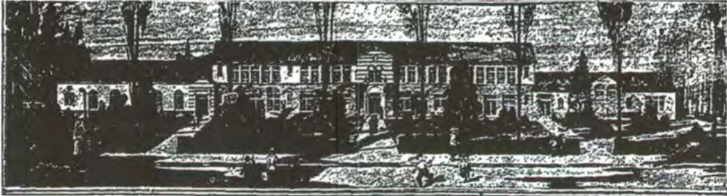
The McKinley School Which is being erected at Chelsea street and Santa Monica Boulevard. It will cost more than $100,000 when complete. Allison & Allison are the architects.
