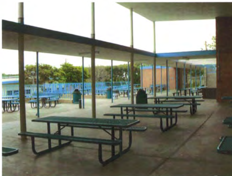
Plate 154. Double Height Porch Over Cafeteria Eating Area (1966-1968)
