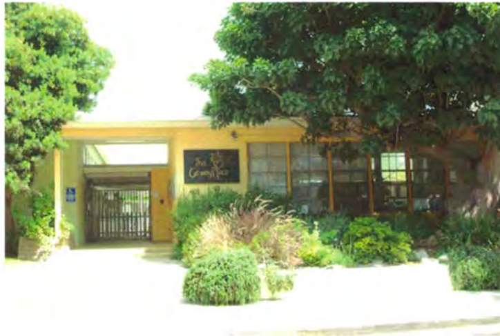
Plate 73. Washington East (The Growing Place), Ashland Street Entrance
