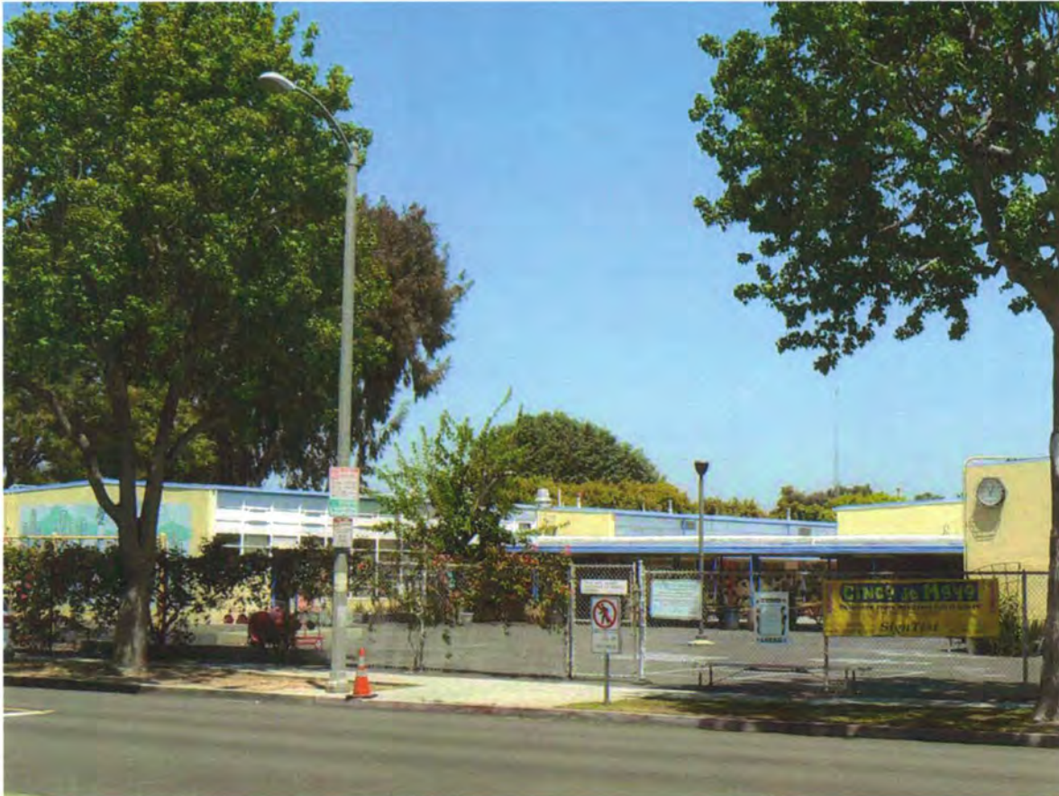
Plate 106. Rear Elevation, Will Rogers School
