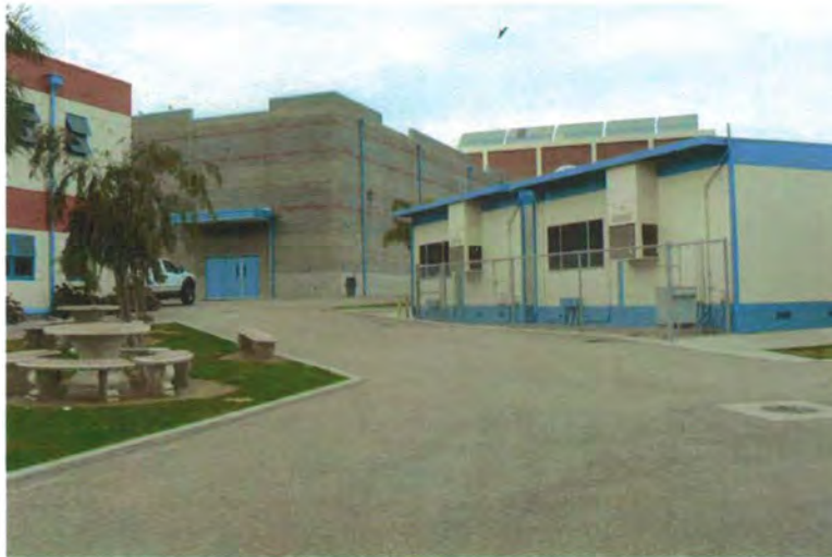
Plate 160. Former Parking Area on West Side of Campus Showing New Classroom (Left), New Gymnasium (Center) and Portable Classrooms (Additions); Original Gymnasium (1968) in Background, View to North
