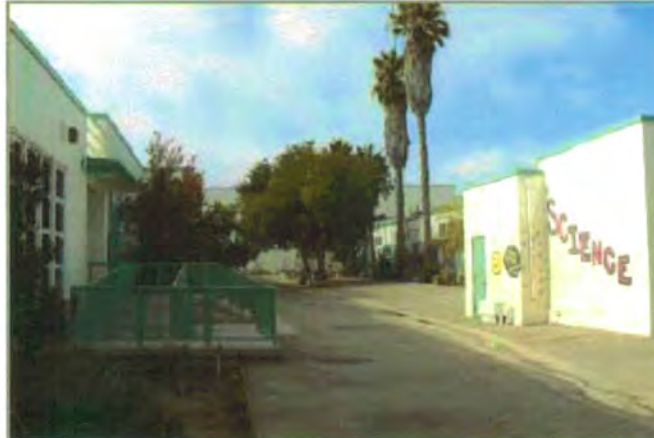
Plate 88. East Campus, Science Building Addition
