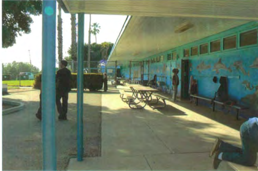
Plate 128. Front Elevation, Original Classroom Building, Cantilevered Overhang
