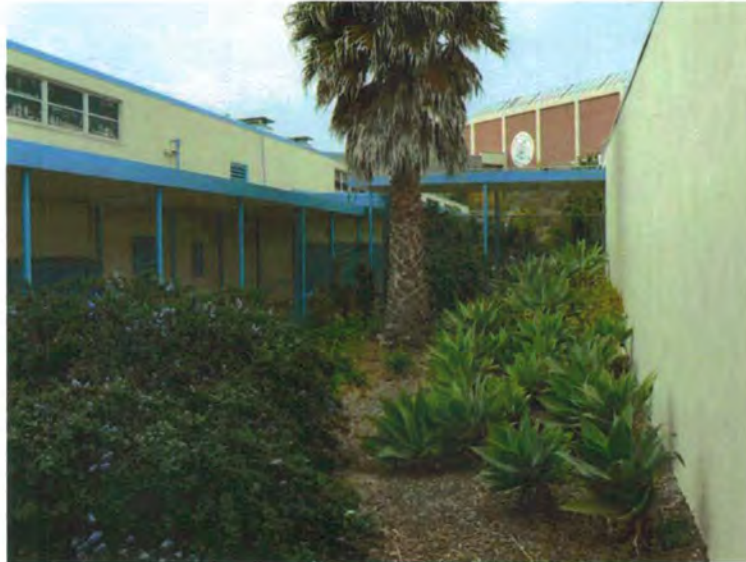
Plate 151. View Toward Original Gymnasium Across Garden Court, to Northeast; Shop Building on Left, Photography Building on Right
