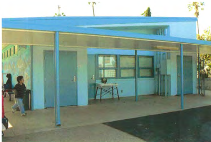
Plate 133. Original Kindergarten, East End Showing Hall Canopy, Slanted and Cantilevered Classroom Roof
