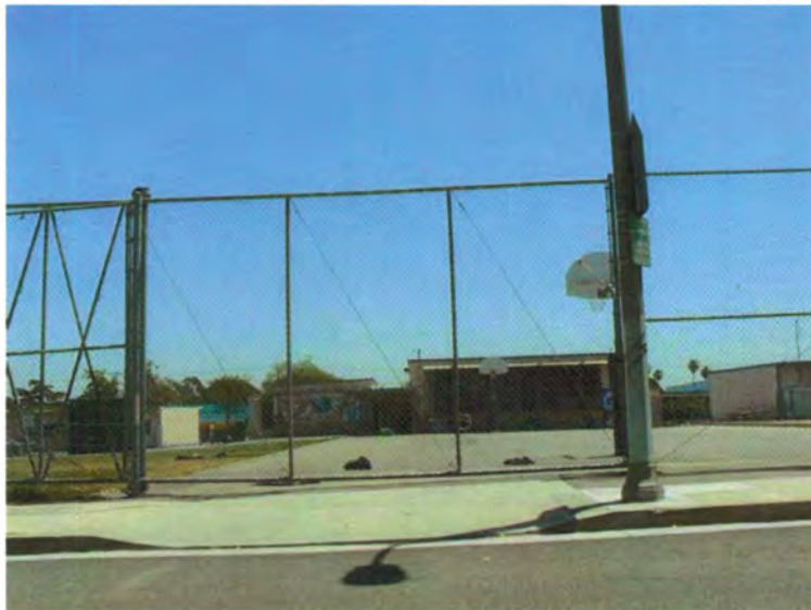
Plate 125. Temporary Classrooms at Rear of School
