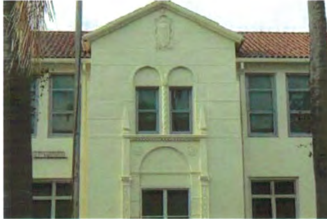
Plate 33. Exterior Architectural Details
