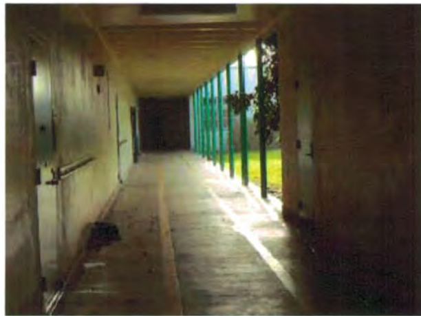
Plate 55. Exterior Covered Hallway
