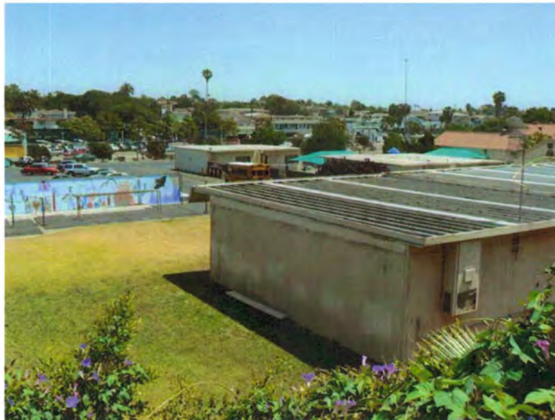
Plate 50. Campus Overview, View to East Showing Temporary Classrooms, Original School in Far Right of Photograph
