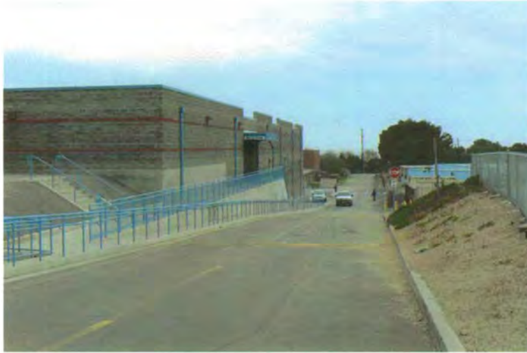
Plate 161. Access Road (Original) Between Malibu High and Juan Cabrillo Showing New Gymnasium and ADA Additions, View to South
