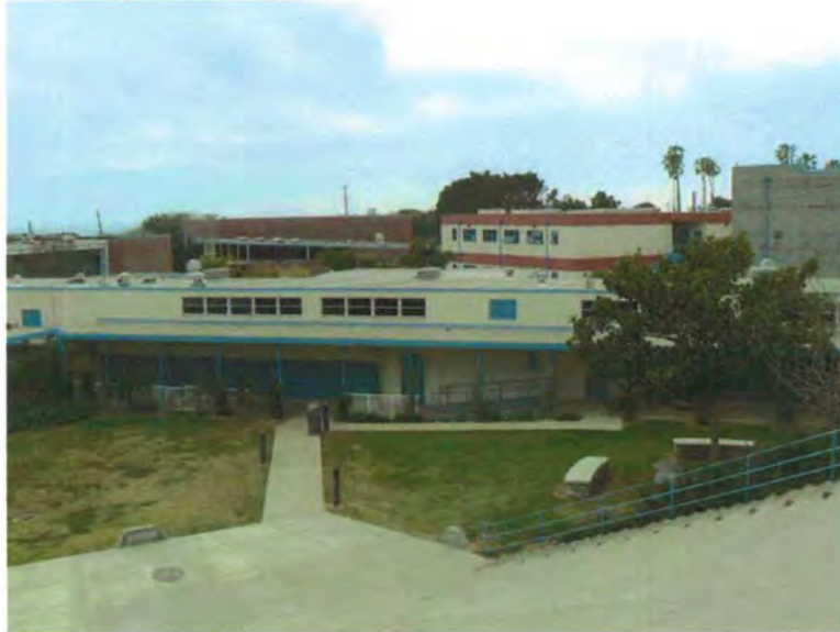
Plate 157. Campus Overview from Amphitheater Showing Shop/Studio Building (1963) in Foreground, Auditorium/Cafeteria in Background (1968), and New Classroom Building and Gymnasium (Additions) in Background (Center and Right), View to Southwest
