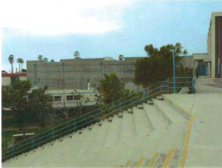
Plate 159. View from Amphitheater Toward New Gymnasium (Addition); Original Gymnasium (1968) on Right, View to West.
