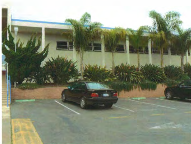
Plate 143. Detail, East Wing Façade, Malibu High
