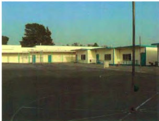
Plate 57. Wing Addition and Temporary Classrooms
