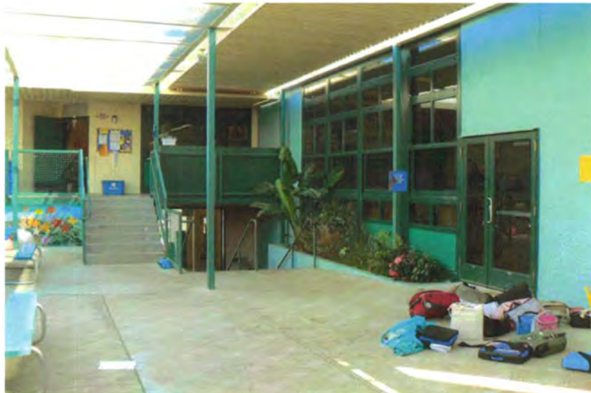
Plate 172. Library and Stairs Down to Playground From Courtyard
