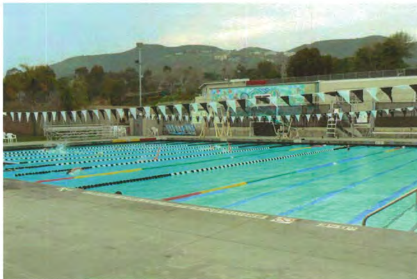
Plate 152. Pool (Enlarged and Renovated), Showing Youth Center (Addition) in Background and Tennis Courts (Original) on Upper Mesa, View to North
