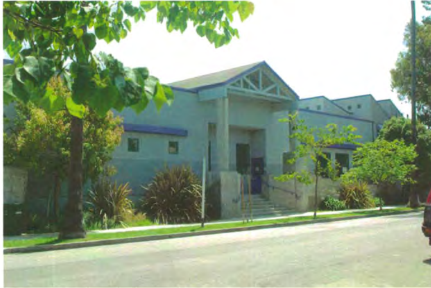
Plate 182. 5th Street Elevation and Entrance Portico, View to Southwest
