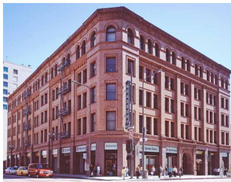
The Bradbury Building in downtown Los Angeles features tan pressed bricks supplied by the Los Angeles Pressed Brick Company. Photo: Library of Congress
