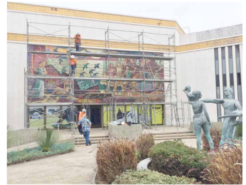
Preparations being made for removal of the mosaic mural on June 17.
