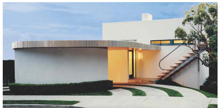
A recipient of a 2018 Stewardship Award, the Entenza House at 475 Mesa Road, is owned by Mike Deasy. Photo: Michael Folonis Architects
