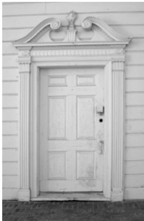
Broken pediment doorway to Marion Davies' old guesthouse at 415 PCH—time-worn but still beautiful.
