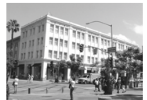
Juniper Building (1912), Third & Santa Monica Blvd.
