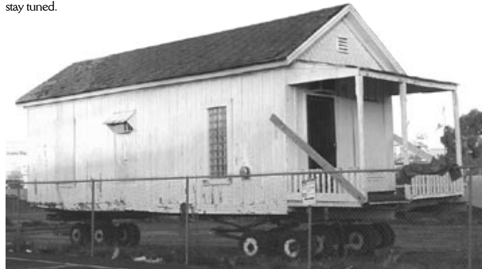
Shotgun House just before the move from Santa Monica Airport
