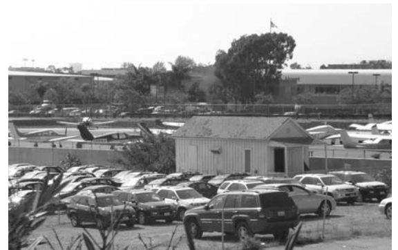
The Shotgun House is safely boarded up at the Santa Monica Airport awaiting a new home.
