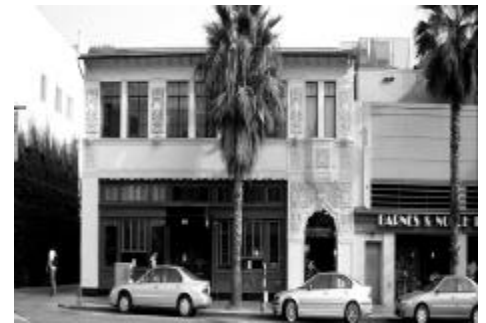
312 WILSHIRE BOULEVARD IS ELIGIBLE FOR LISTING IN THE NATIONAL REGISTER
