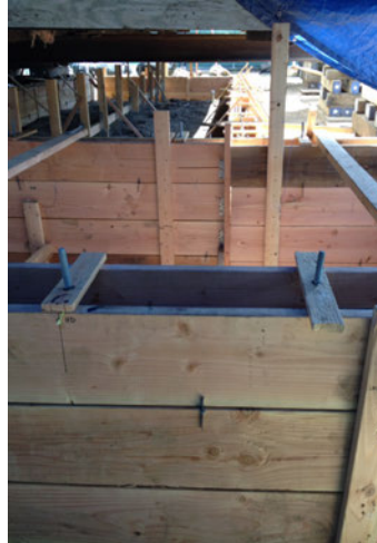
Wood forms were built to form the concrete.
