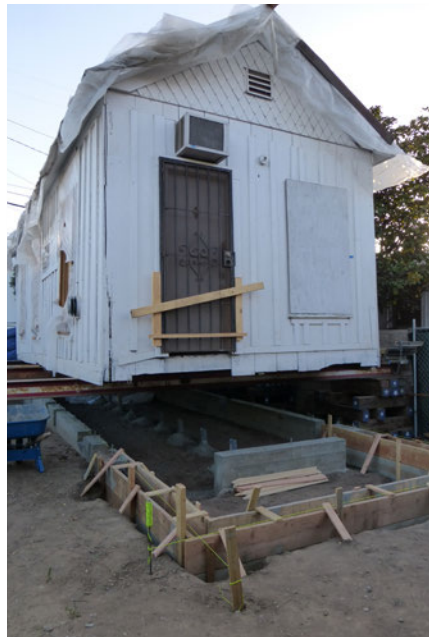
Here is the house with the forms in place for the front porch foundation. By publication of this newsletter, the Shotgun House will have been lowered into place on its new foundation.
