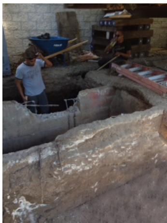
Here is the house with the forms in place for the front porch foundation. By publication of this newsletter, the Shotgun House will have been lowered into place on its new foundation.
