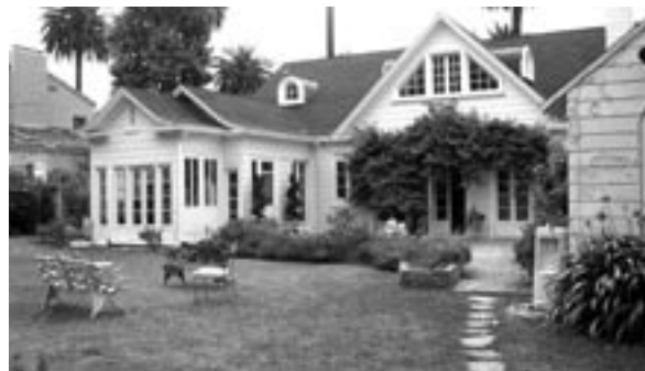
Rear view of the Farquhar House now under renovation.
