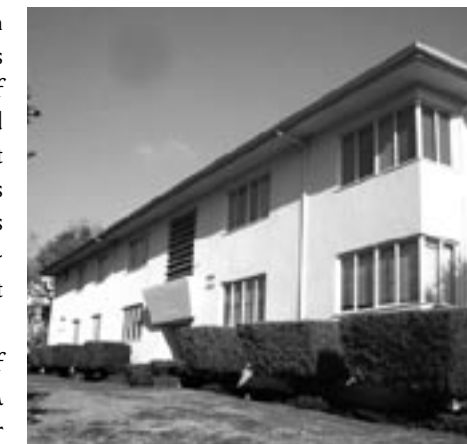
Garden apartments reflect the city’s mid-Century growth.
