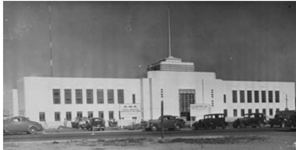
Santa Monica City Hall under construction 1940. Note the P.W.A. sign just left of center. Photo courtesy of the Santa Monica Public Library Image Archives.
